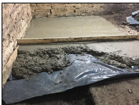
IMPROVEMENTS have been made to the basement at the VIC Centre so that it can be used in future. A new floor has been laid, thanks to Simon Peace and Andy Greaves, which will enable the space to be used by the centre.
