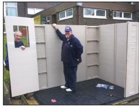
"The original shed had been removed but the base was still there so we had to do some digging and levelling of the ground and we laid some flags for the new shed.
